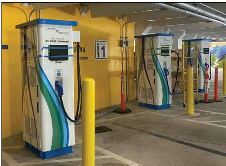
New EV Charging stations being installed in Thunderbird Parkade.
