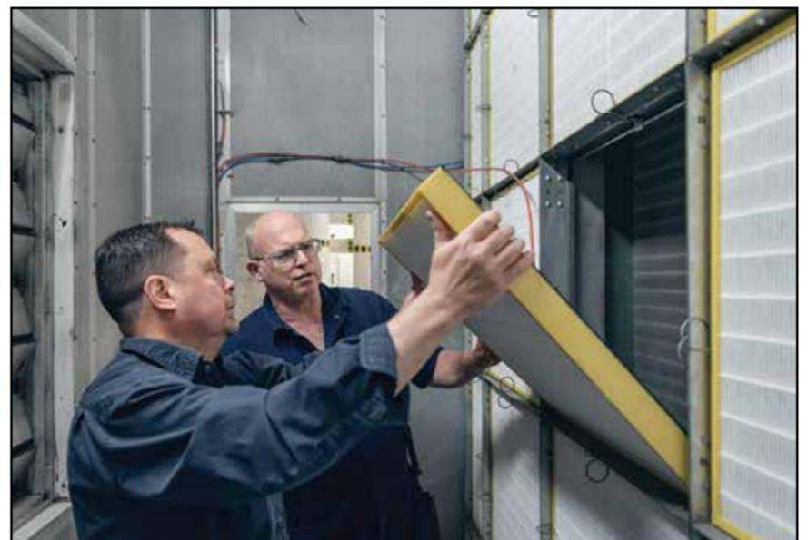
Shawn Kenney (left) and William Guest (right) from UBC Vancouver changing the MERV 13 air filters in an air handler unit located in the Pharmaceutical Sciences Building. Photo credit: UBC
