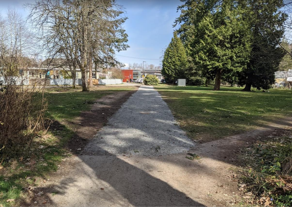
The above image shows the work done in 2021 to connect to Norma Rose Point east of the Acadia Park walkway (looking east to Norma Rose Point School). The planned works will match this pathway, but with smaller crushed gravel for easier cycling, particularly for smaller children.
