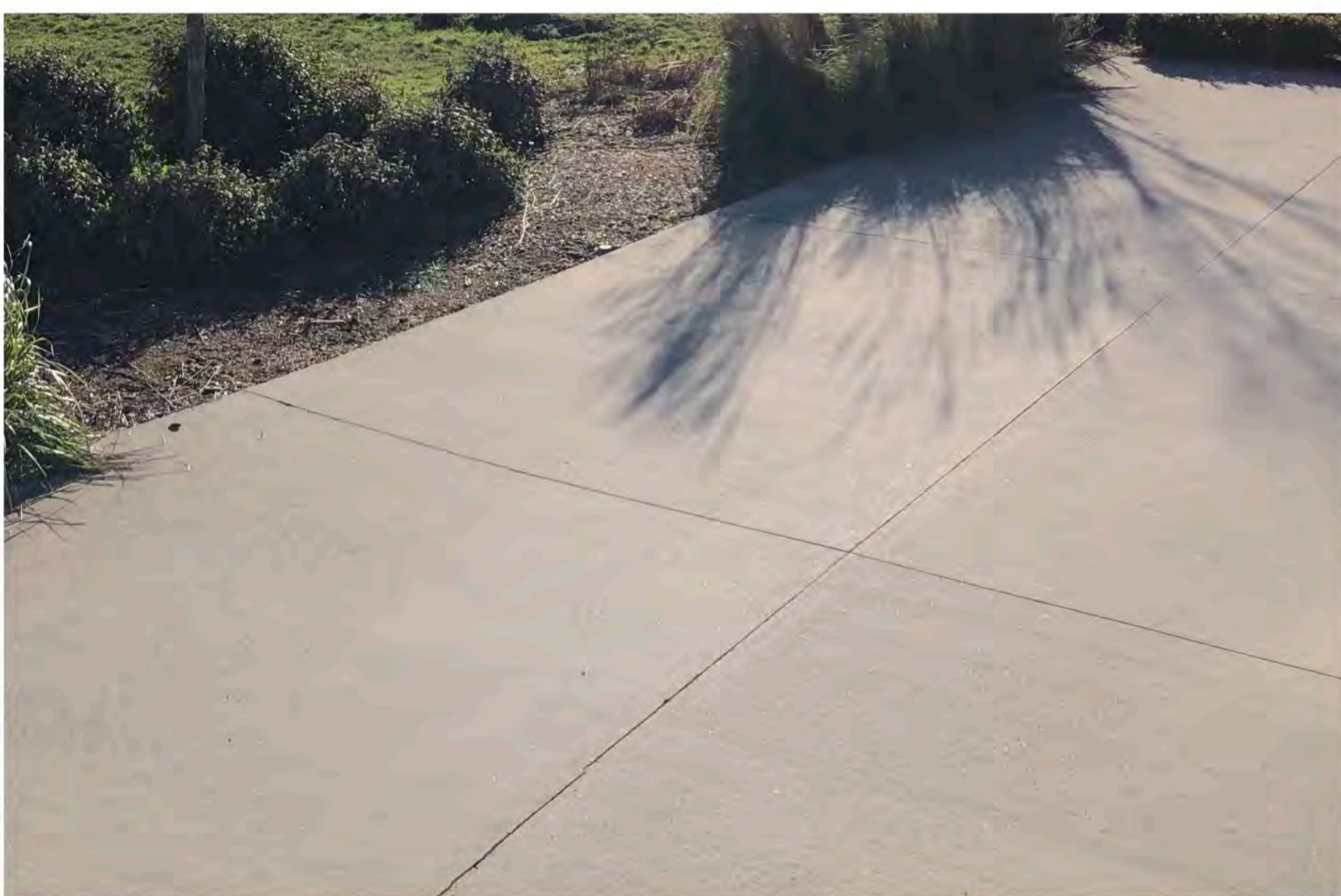
Reference Images-CIP Concrete with Light Broom Finish; in-keeping w/ UBC Standards and Tech. Guidelines and current Park Detailing
